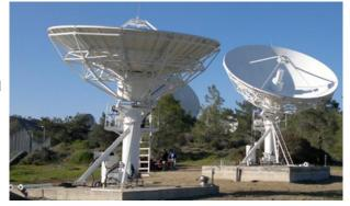
CSM, although simple in its concept, can become complex when it involves multiple satellite transponders from multiple antennas. Extensive cabling, LNB power supplies and controls, slope compensation and signal management is needed to ensure that the satellite signals reach the Signal Analyser sub-system with the right C/N and signal level to be useable for the application.
